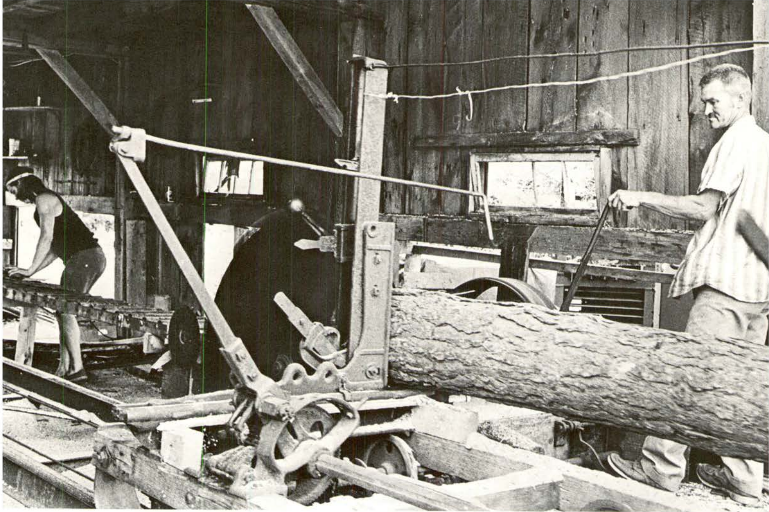
About 770 of 1,700 wood industry jobs are directly dependent on the wood cut in Tug Hill.
