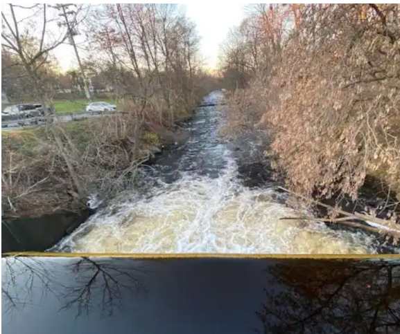
Downstream conditions directly above Little Salmon Dam (Fall 2025) [left]. ←
