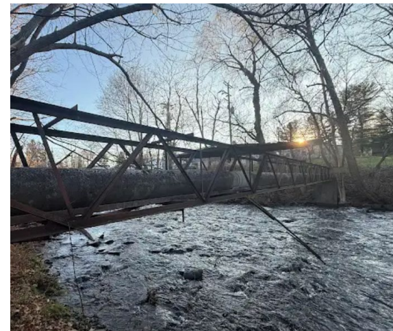
Gravity fed sewer main downstream (Fall 2025) [right]. →
