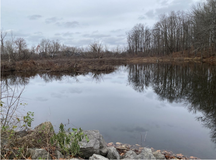
Upstream conditions directly above Ames Mill Dam (Fall 2024).
