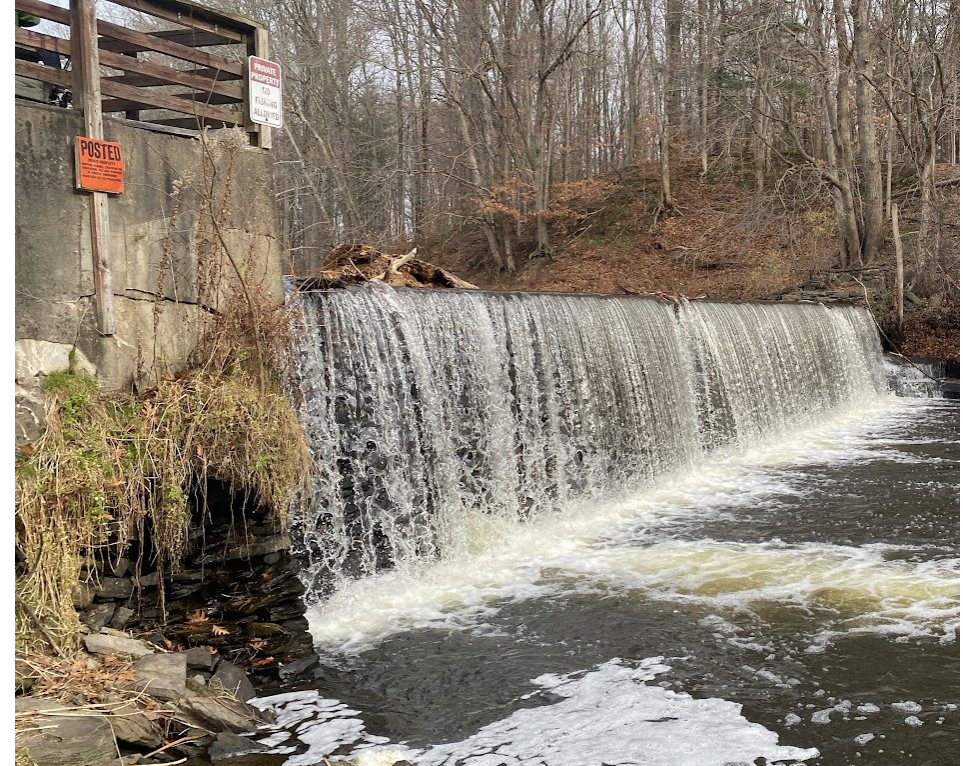
Ames Mill Dam in Village of Mexico, NY (Fall 2024).
