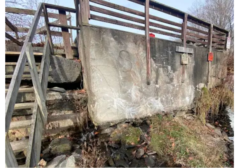
Concrete structure on inner bend of the Ames Mill Dam (Fall 2024).
