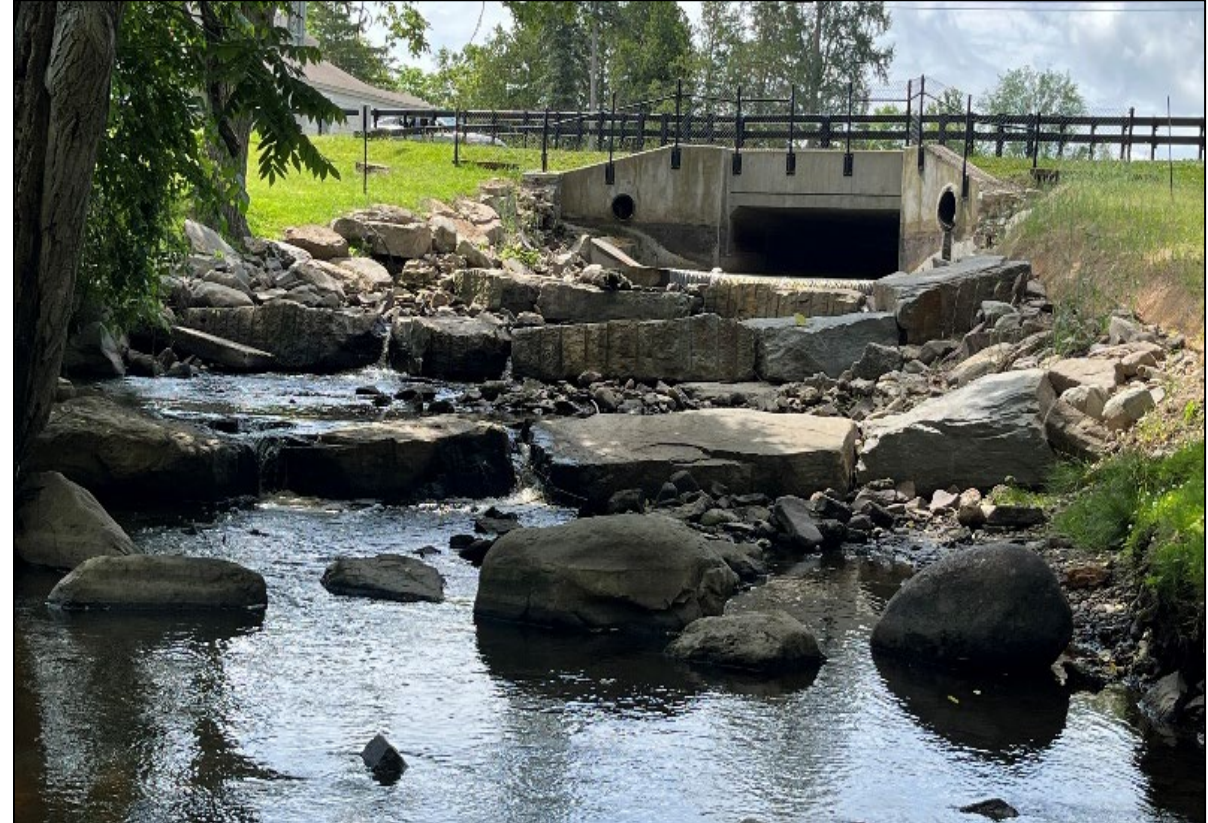
Re-Engineered Step-Pool Design
