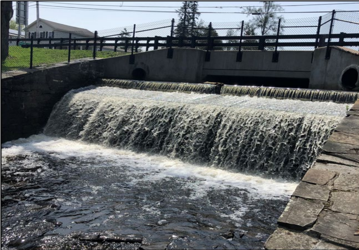
Original Dam Structure
