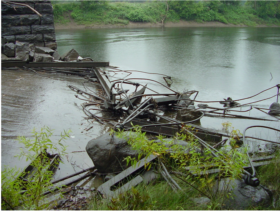
Photograph 7. Old Whittlesley Bridge remnants.
