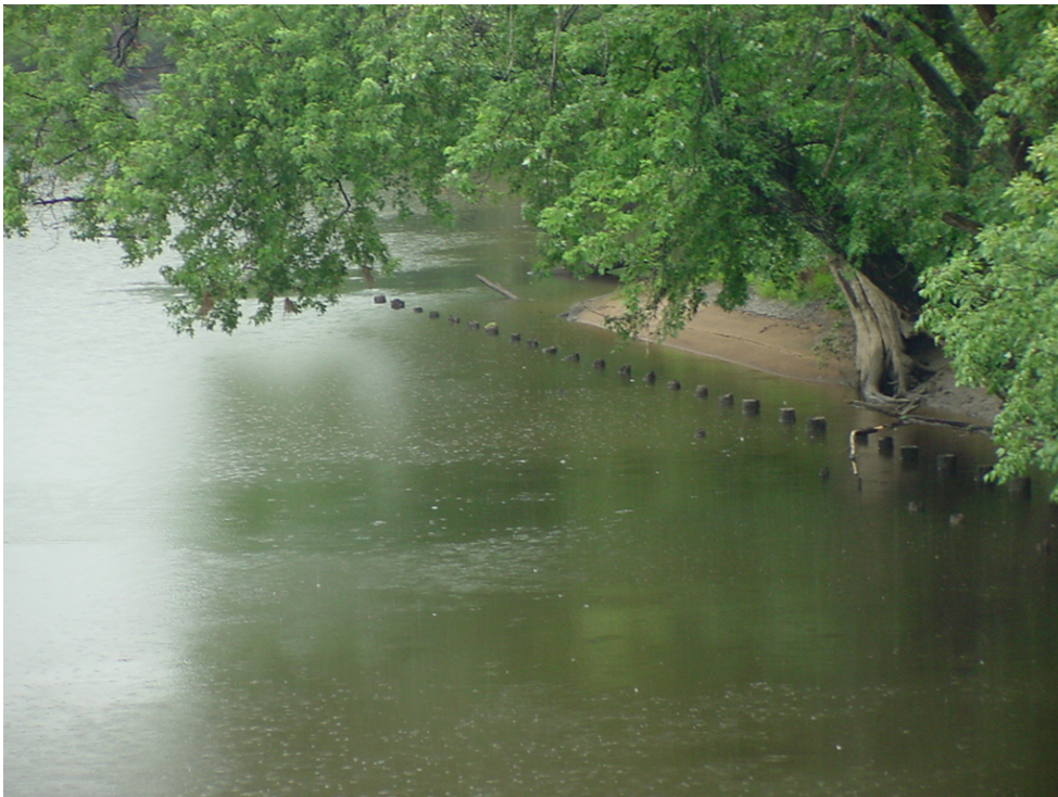
Photograph 12. Number 4 Road Bridge (Site 14).
