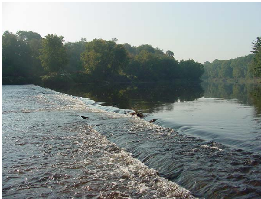
Photograph 2. Jetty Dam below First Creek with timbers and metal spikes (Site 2).
