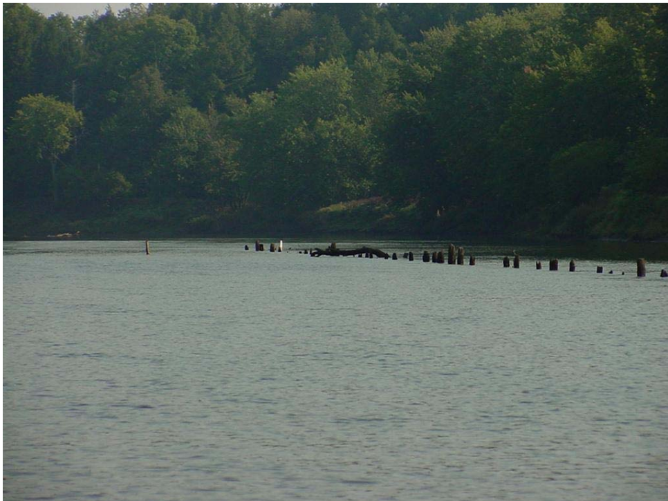
Photograph 8. Timber piles below Whittlesley Bridge (Site 6).
