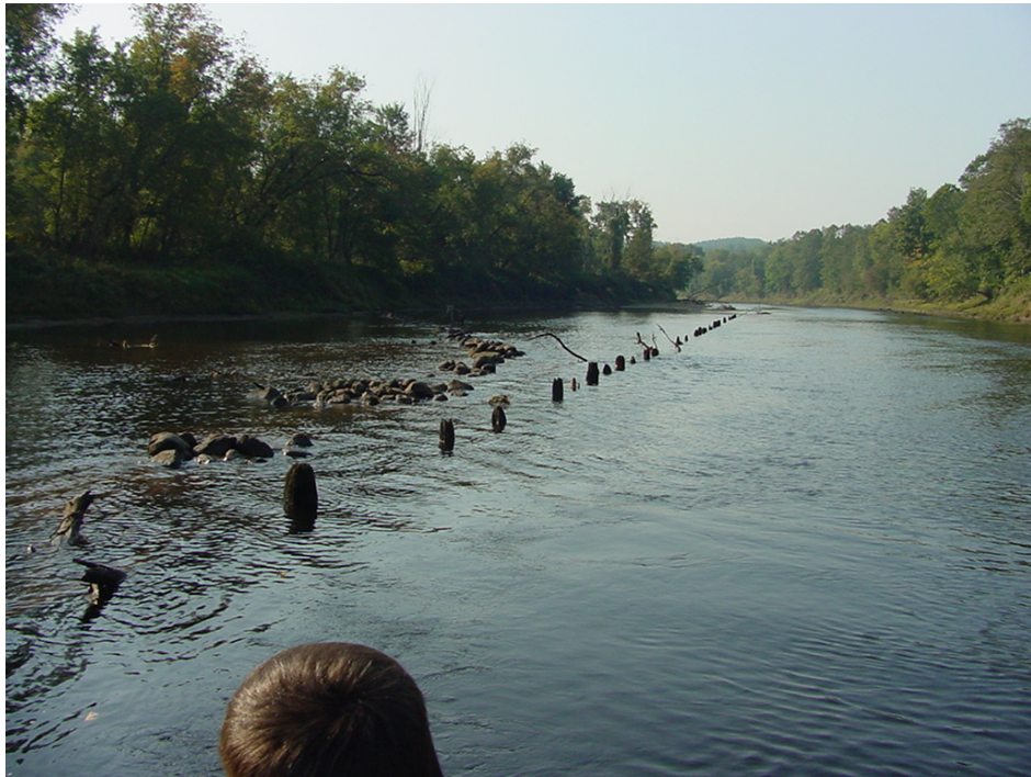
Photograph 5. Timber piles with rock jetties (Site 4, looking south).
