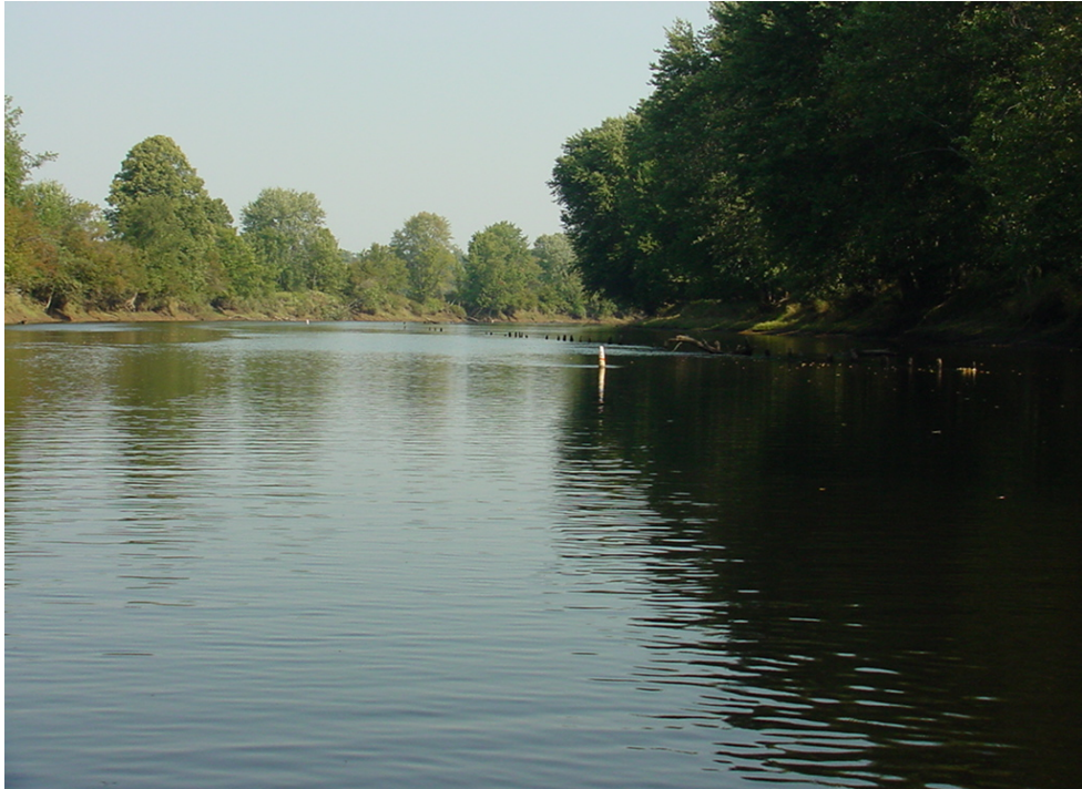
Photograph 9. Timber piles with buoy (Site 9).
