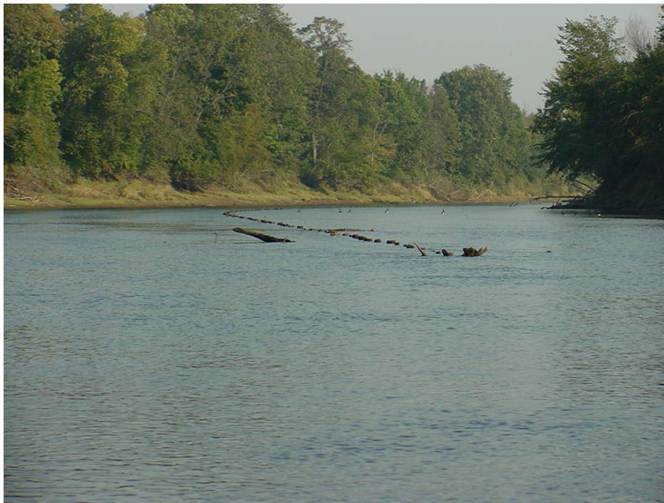
Photograph 4. Timber piles and former training structure (Site 4).
