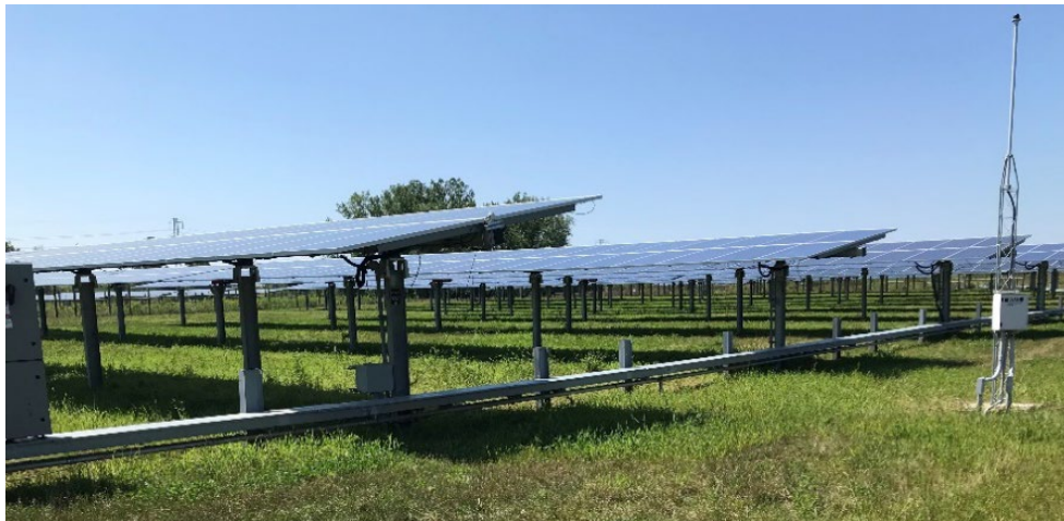
Solar installation in Seneca County which shows the above ground infrastructure, which could present problems for mowing or sheep grazing. Photo: Joe Lawrence
