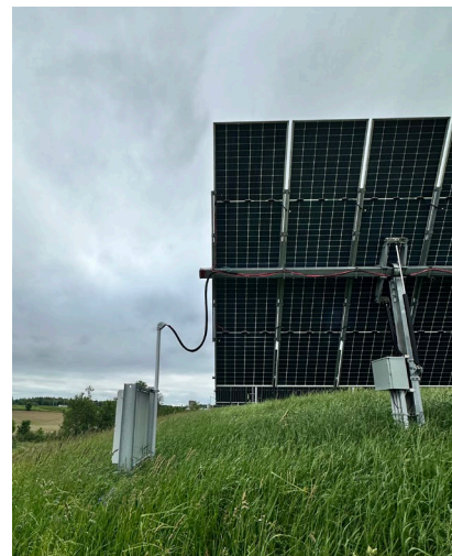
Two-panel portrait (2p) configuration at the ClearPath Energy New Bremen One site.
