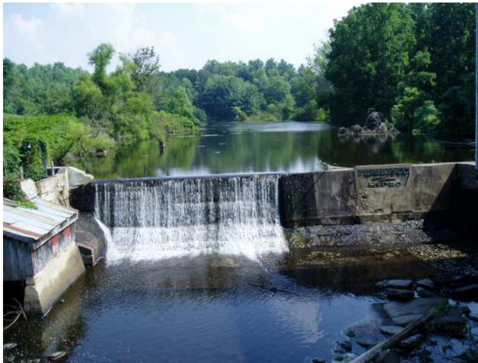
Figure 11. Fernwood Dam, Grindstone Creek, Fernwood
