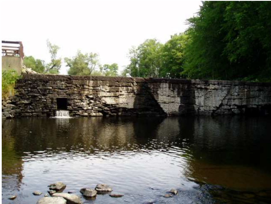
Figure 7. Ames Mill Dam, Little Salmon River, Mexico
