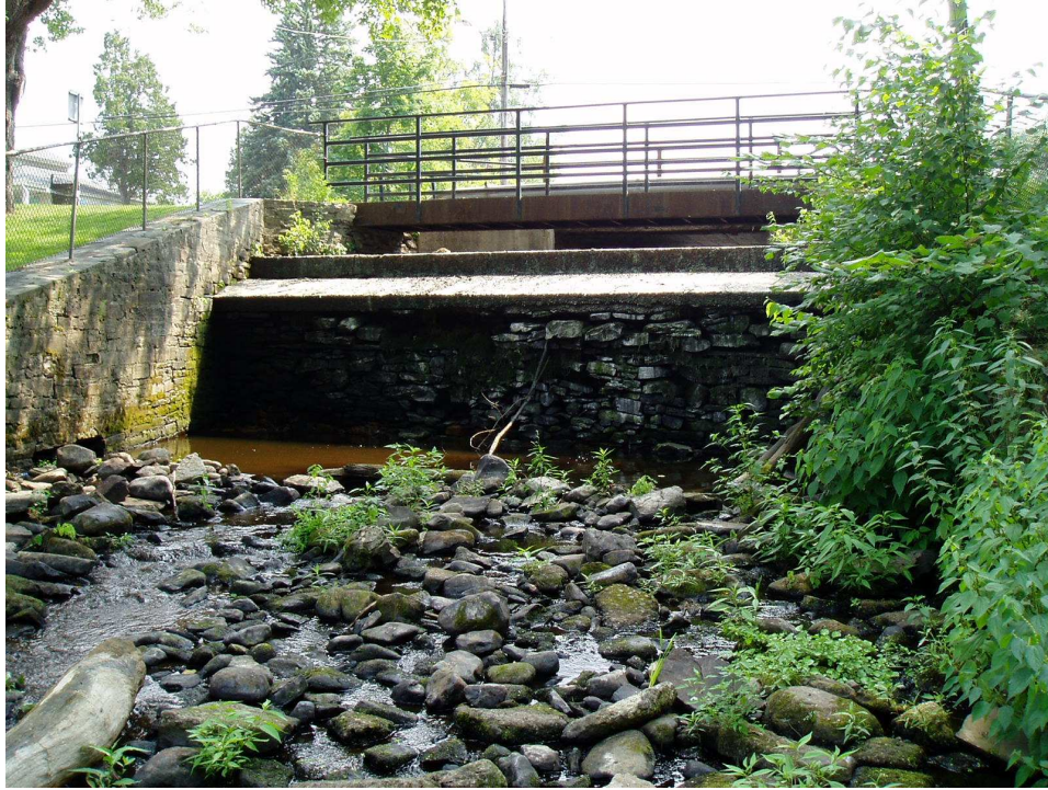
Figure 5. Youngs Mill Dam, Black Creek, Mexico
