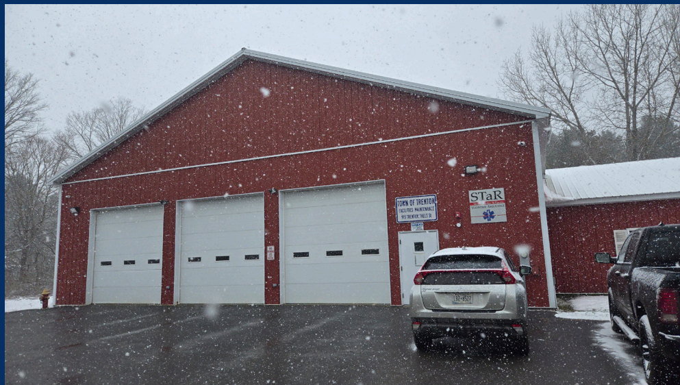
STaR Volunteer Ambulance Facility, Prospect, NY
