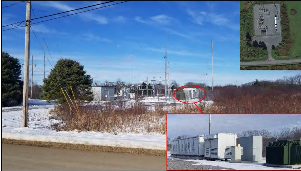
The Pulaski small, 2 MW battery energy storage system, designed to sustain a 2,000-kW customer demand, as seen from the road. The top right portion of the image shows an aerial view of the storage system (source: Google Earth Pro). The bottom right portion of the image shows the storage system up close (source: NYS Tug Hill Commission).
