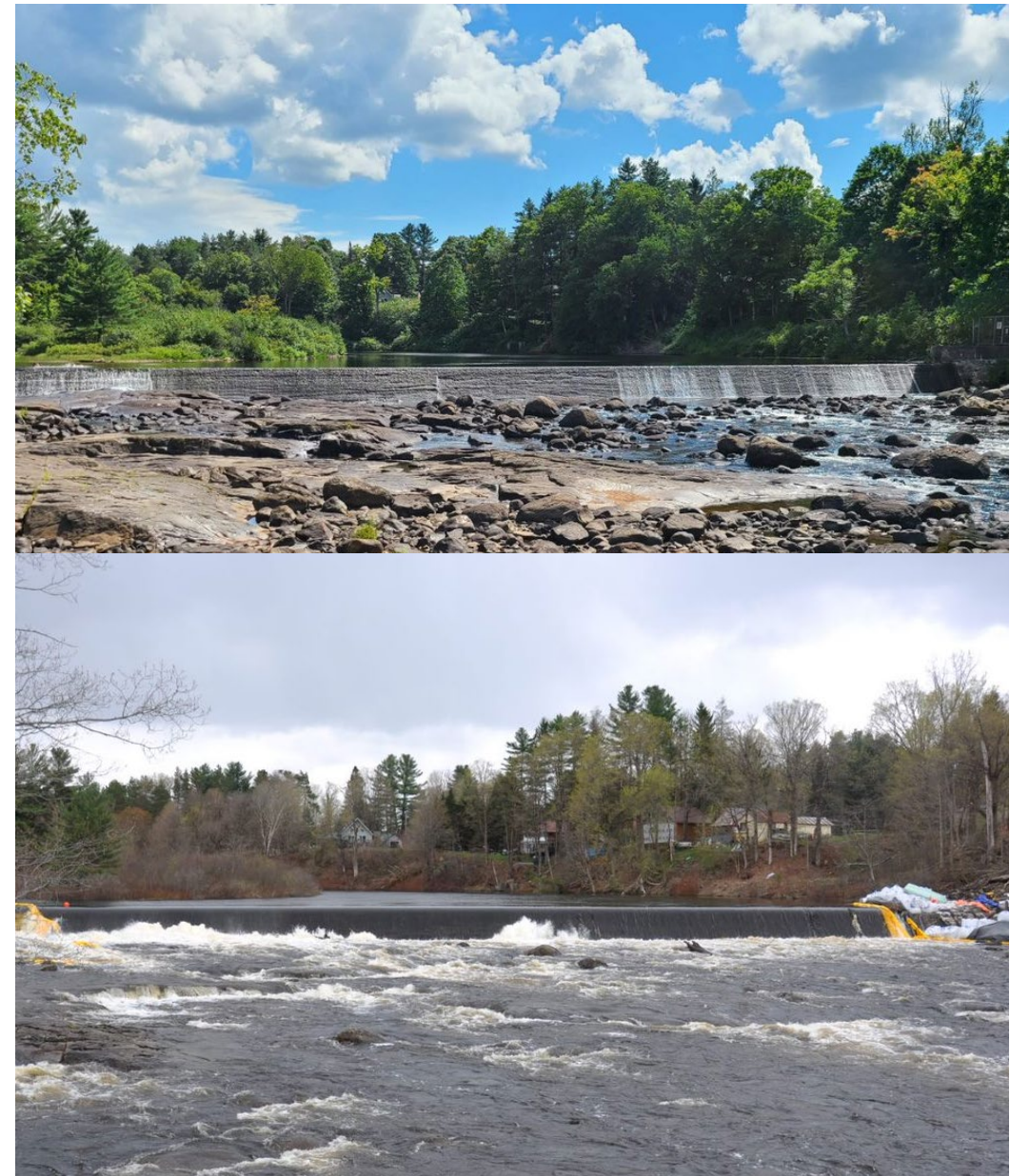
Hawkinsville Dam, summer of 2022 (top) and spring 2023 (bottom)
