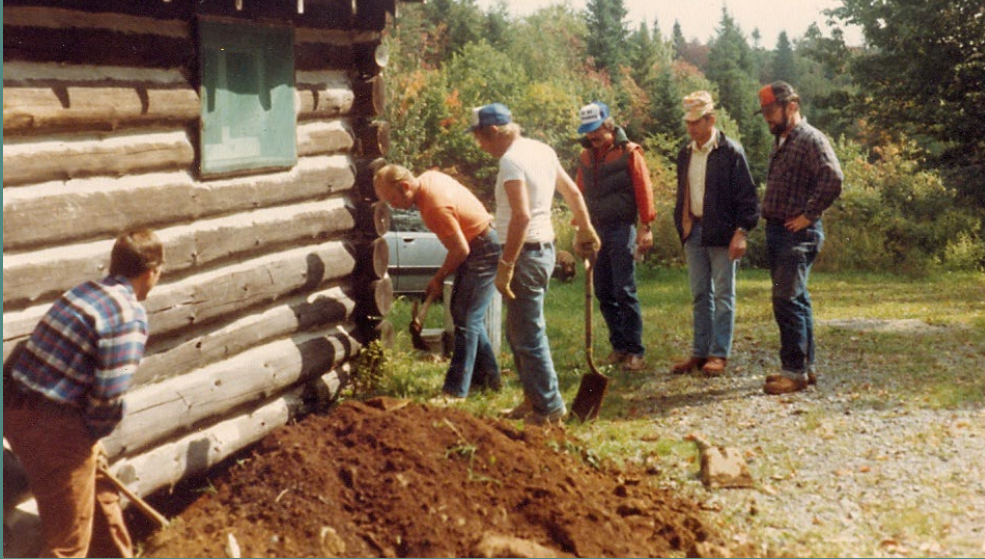
Repairing/preserving bottom log, September 20, 1981.
