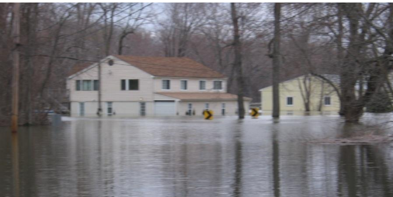
Moderate flooding - Connecticut River at Portland, CT.
