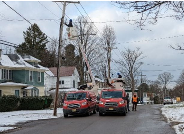
Crews installing new LED streetlights in Carthage.
