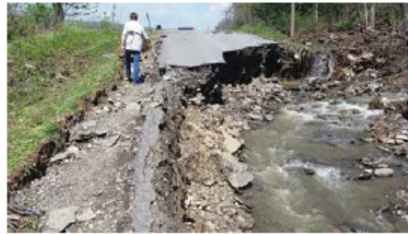
East Valley Road, north of Branchport, NY. Floodwaters were beyond the capacity of existing ditches and culverts. Many area roads were damaged from the velocity and volume of the floodwater. Photo: Courtesy of Dave Enty (NWS Binghamton).
