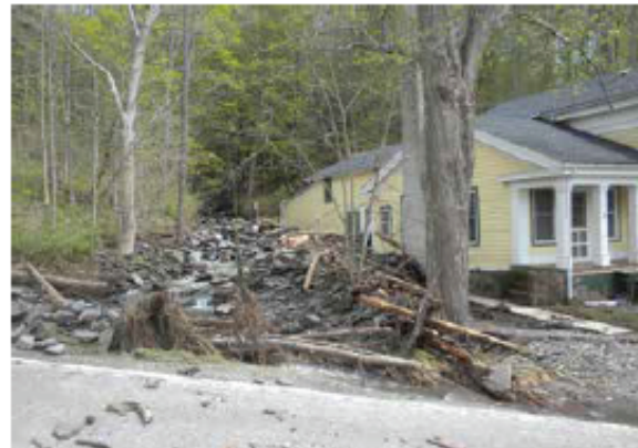
As floodwater travels across the land, it picks up debris. This house was nearly surrounded by debris that was left from receding floodwater. Photo: Mary Austerman, New York Sea Grant.
