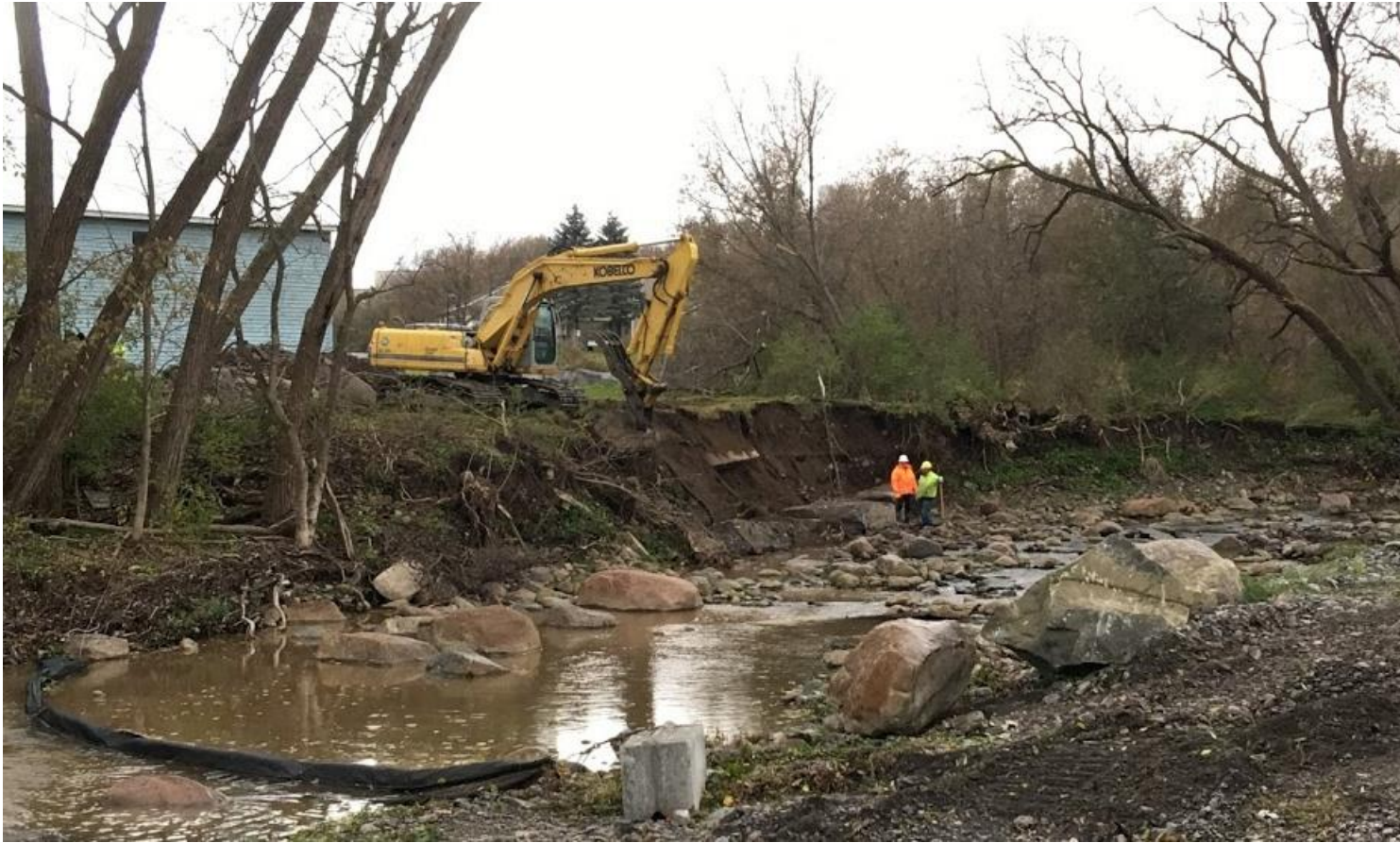
Protecting private and public infrastructure in Lowville along the Mill Creek
