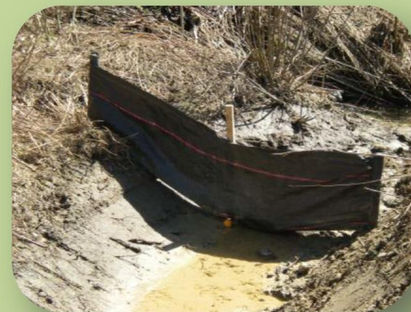
WRONG! An example of an ineffective erosion control practice – silt fencing should be buried to a depth of about 8 inches
