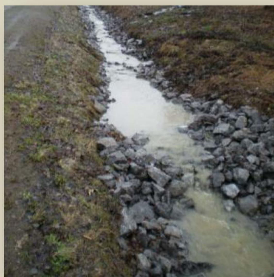
Rock-lined ditches and check-dams are a cost-effective technique for reducing runoff from roads and ditches
